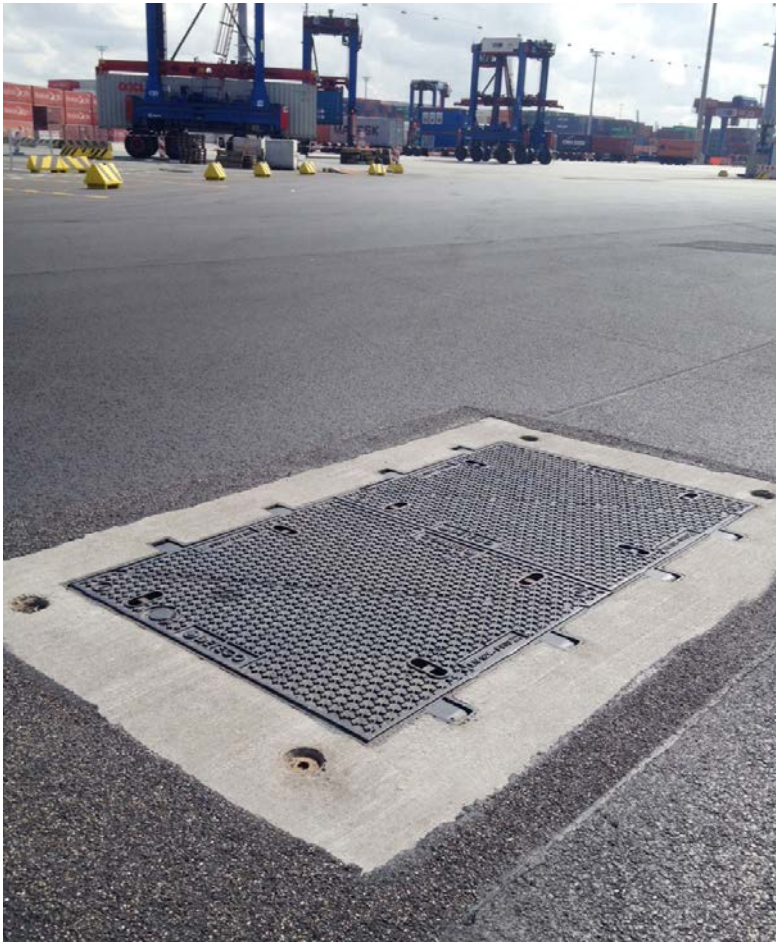
Cast-iron cover with triangular covers, prefabricated concrete frames, load class F 900
