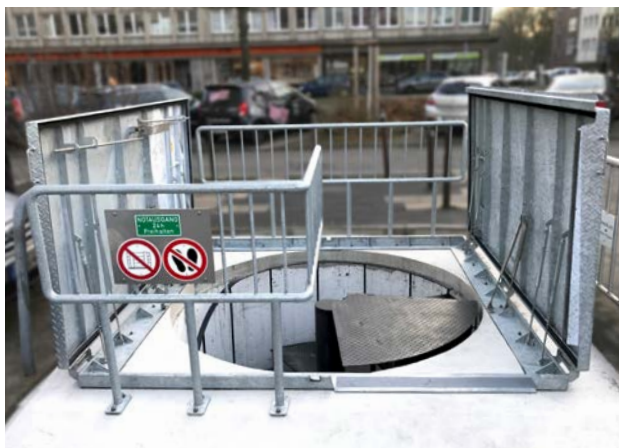
Escape hatch cover, safe to walk on, can be operated manually, Essen
