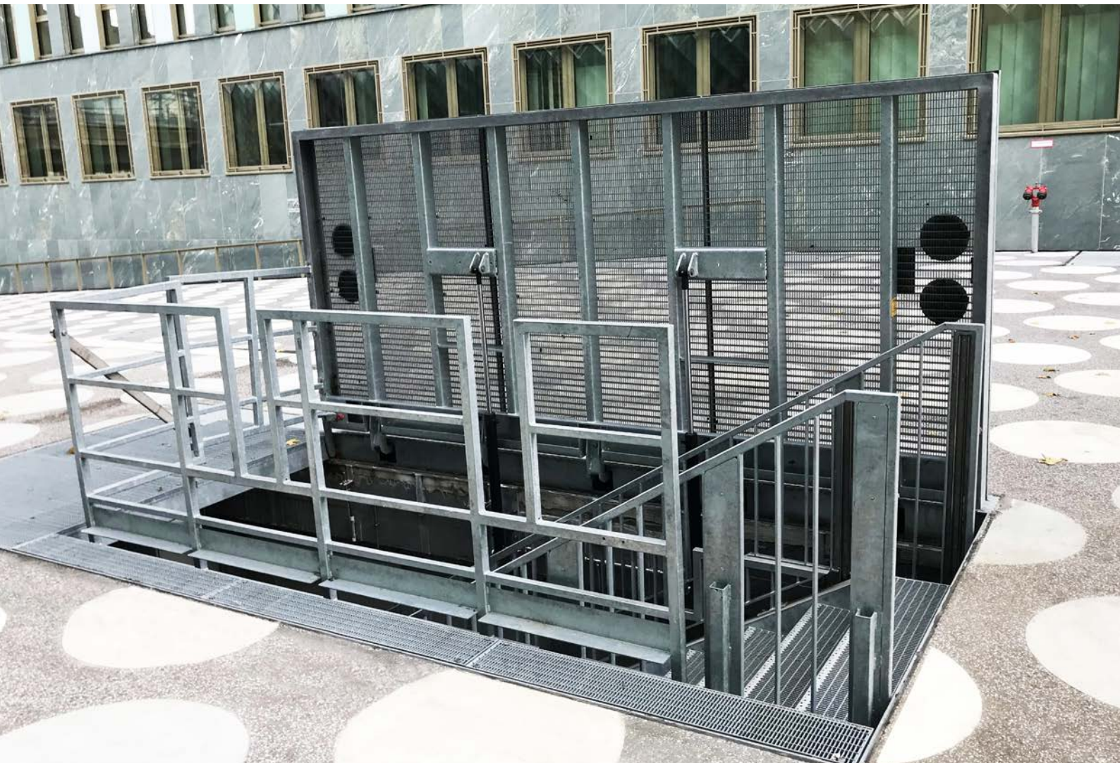
Floor gate and emergency exit at Berlin's Futurium future museum in the immediate vicinity of the Reichstag and the main railway station: The escape staircase including handrail is fully extended and accessible within 25 seconds
