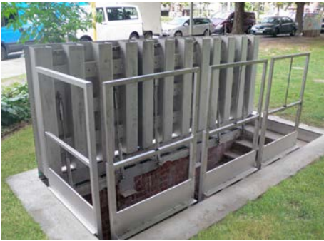
An opening aid provides assistance to manually opening the cover
