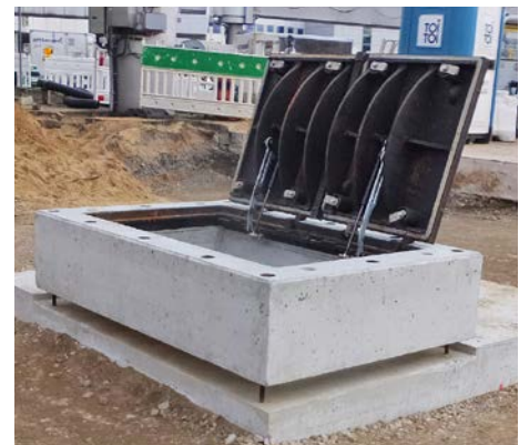
Prefabricated surface-water-tight cable shaft cover with a height-adjustable reinforced concrete frame, Düsseldorf
