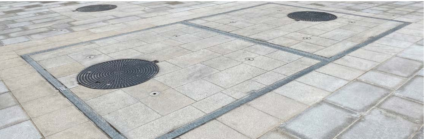
Underground railway station with entry and exit openings for smoke extraction technology and inspection openings for quick access, Karlsruhe city centre
