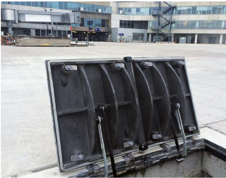
Surface-water-tight cable shaft cover, reinforced concrete frame, class F 900, Frankfurt
