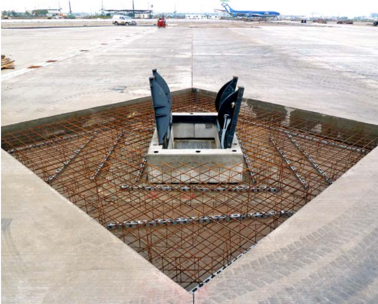
Prefabricated triangular cable shaft covers with a height-adjustable reinforced concrete frame and a load class of F 900, Frankfurt
