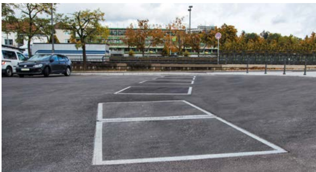
Backwater-proof covers filled with asphalt and with a load class of D 400, Ansbach
