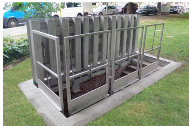
Three-piece cover with opening aid and folding guardrail, Frankfurt
