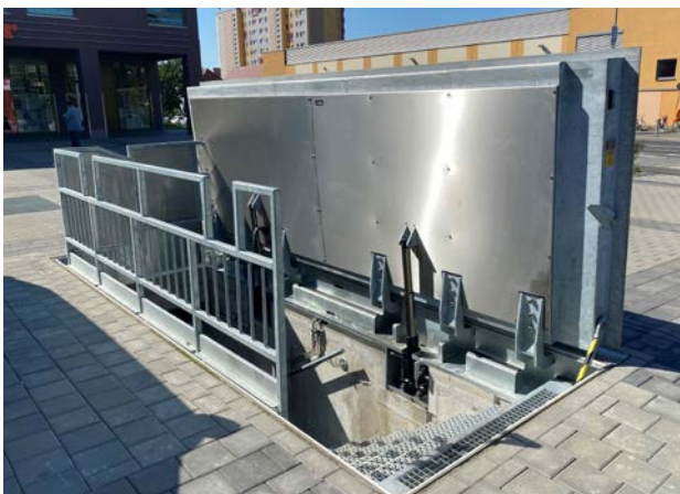
Hydraulic escape hatch with collapse protection, Berlin
