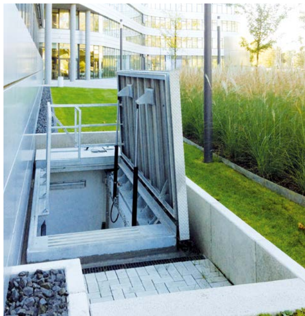
Hydraulic stainless steel escape hatch, Cologne
