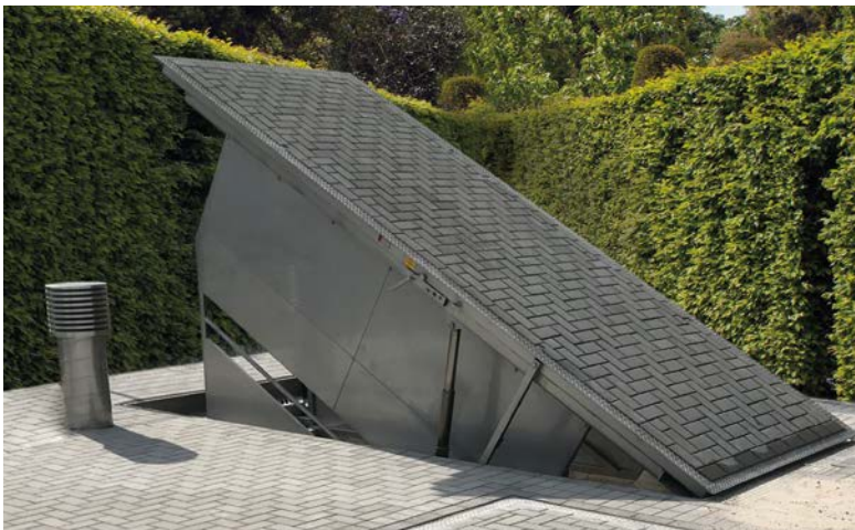
Pump station access, Seligenstadt
