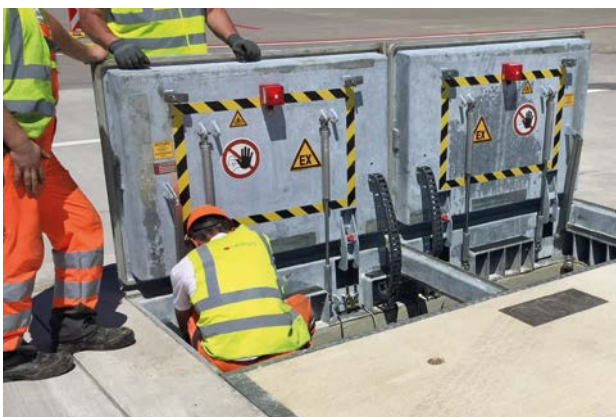
Heavy load cover with two inspection openings, load class F 900
