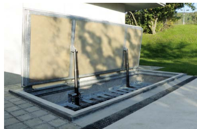
Hydraulic cover on a woodchip silo with a fire protection classification of F90, Eisenstadt/Austria
