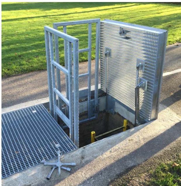
Escape hatch with a telescopically retractable grating, Leverkusen
